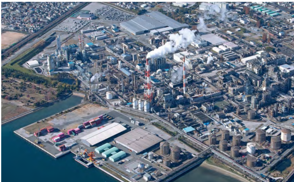
Aerial photo of Aboshi Plant, Himeji Production Site, Daicel Corporation
