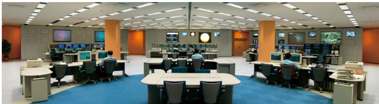
Control room of the Integrated Production Center (IPC), at the Aboshi Plant, Hyogo Prefecture
