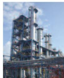
The Company's Ohtake Plant began operation of Japan's first ethyl acetate manufacturing facility using the ethanol method. This facility boasts an annual production capacity of 50,000 tons. Ethyl acetate has wide-ranging applications, including uses in inks, paints and pharmaceutical and agricultural chemicals, and demand is expected to grow as the substance replaces toluene and provides for many other useful applications.
